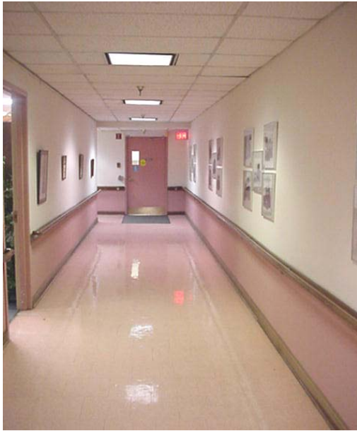
Condition before renovation
