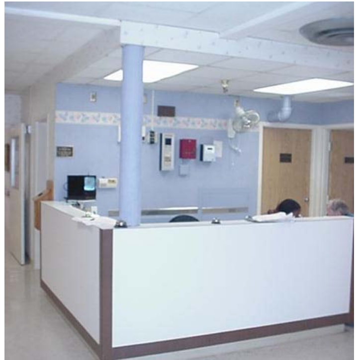
Nurse Station before renovation
